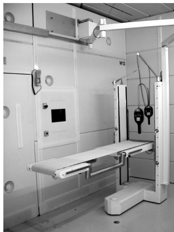
Fig. 7. Irradiation room with treatment couch. The fixed horizontal beam enters from the left, 1.45 m above the floor.
